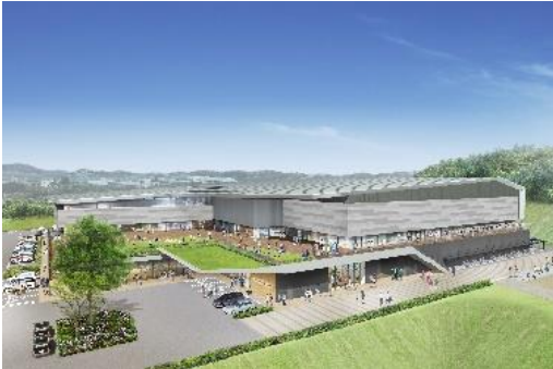
Project for construction of a new gymnasium, Shiga Prefecture
