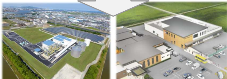
Biomass resource reuse facility in Toyohashi City
